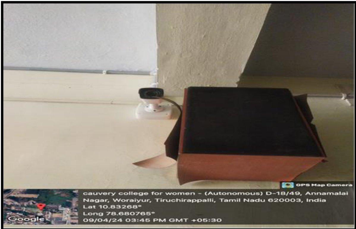
HOSTEL – A BLOCK SECOND FLOOR
