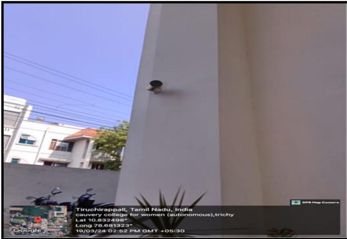
A – BLOCK GROUND FLOOR ENTRANCE - RECEPTION CAMERA
